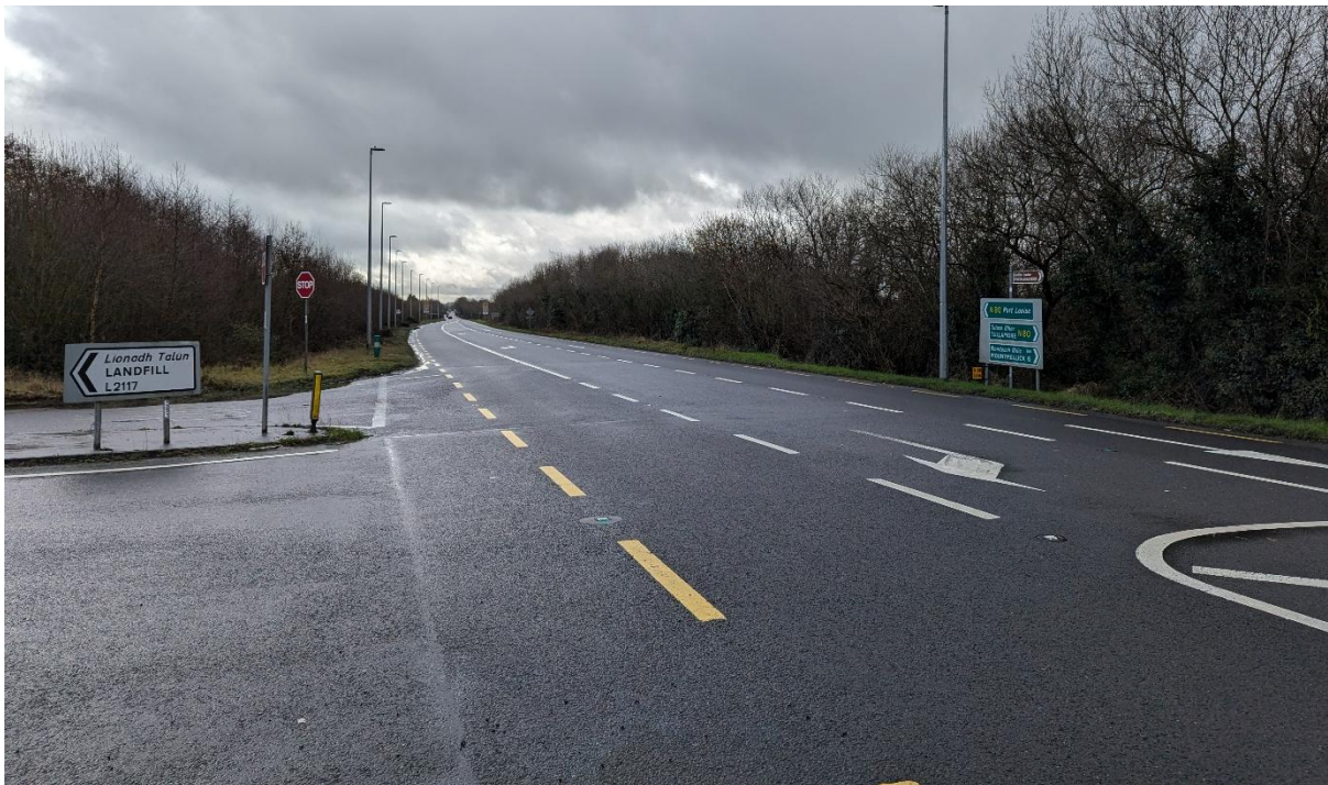
Figure 13.6: N80 (Facing south)
