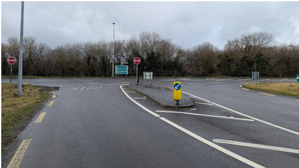
Figure 13.7: Junction N80/L2117 (Facing west)
